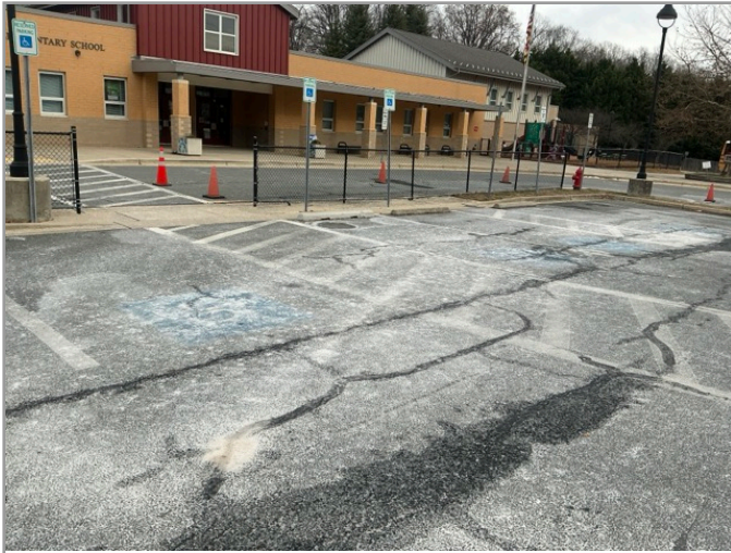
OVERVIEW OF ACCESSIBLE PARKING AREA
