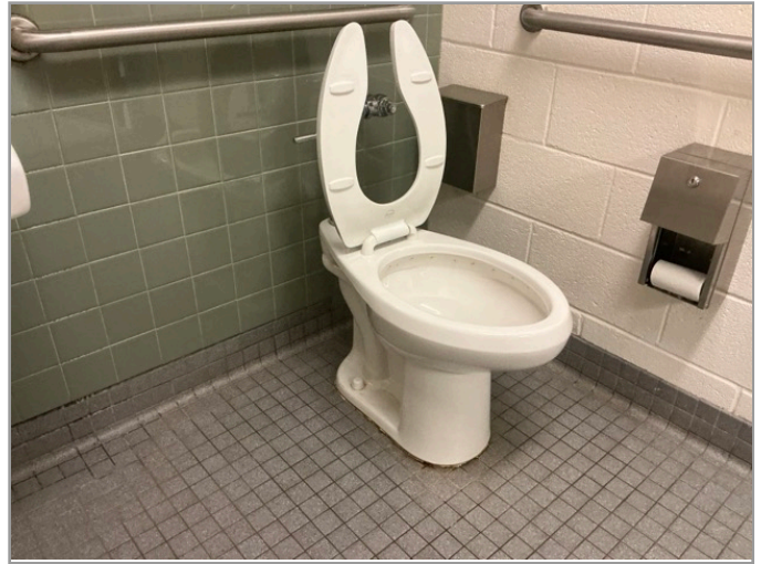
TOILET STALL OVERVIEW
